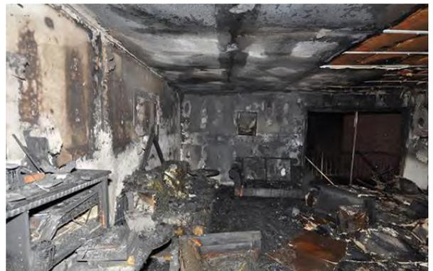
Above, images of the fire scene where a firefighter in Maryland lost his life. The two images show the difference in smoke and fire damage to a room where the door was left open (first image) and closed. These apartments were side by side. Photo Sourced from ATF FRL
